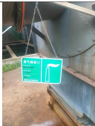
DA001 排放口标牌
