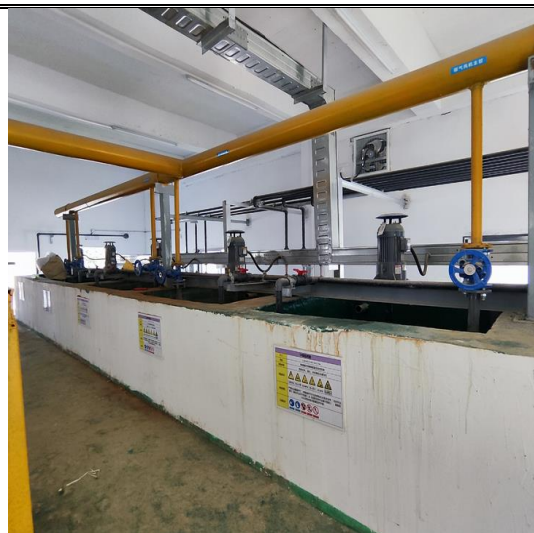
污水站加药区防腐防渗
